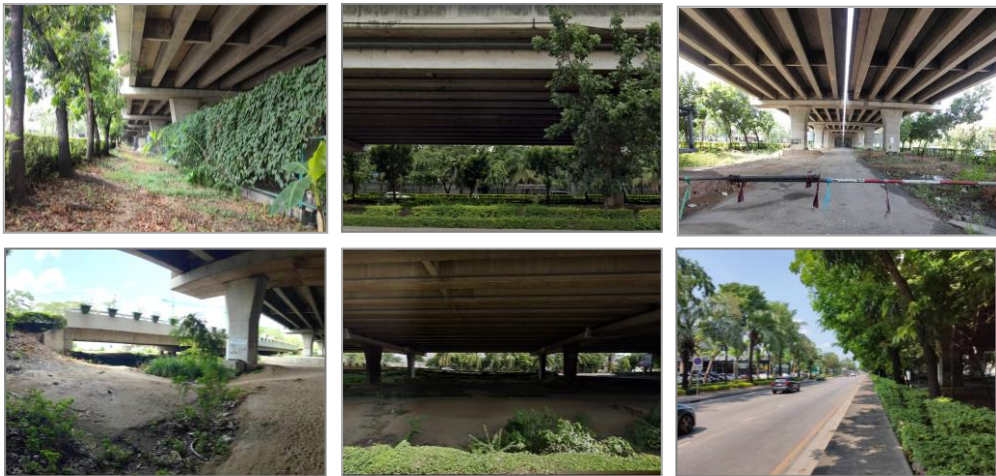
Figure 3 - 8 Images of the site.
