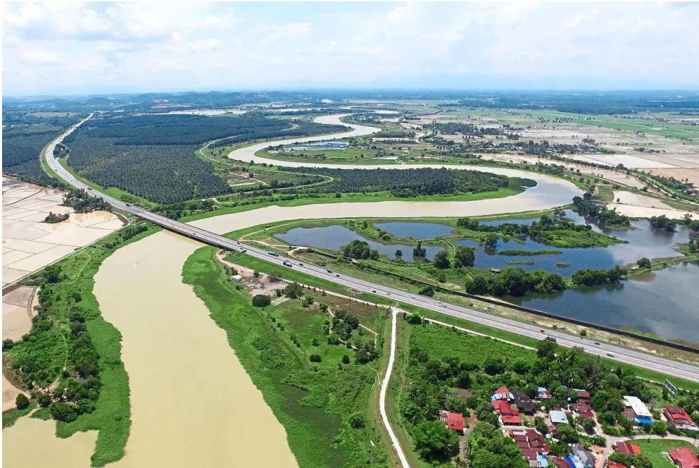
Figure 1 Sungai Muda , Kedah, Malaysia
