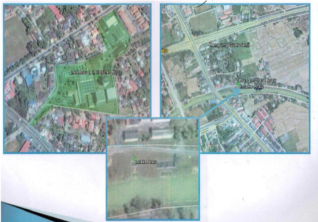
Figure 4 Arau Water Treatment Plant I-III
